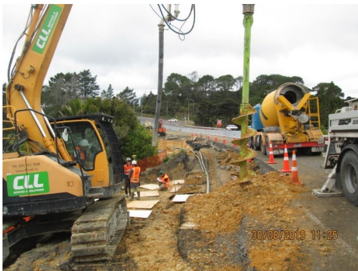
Work on retaining structures at Dairy Flat Highway intersection with Coatesville Riverhead Highway
